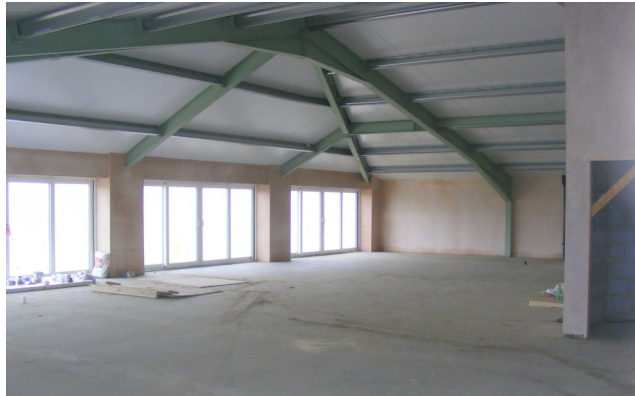
First floor, now with floor and plaster walls
