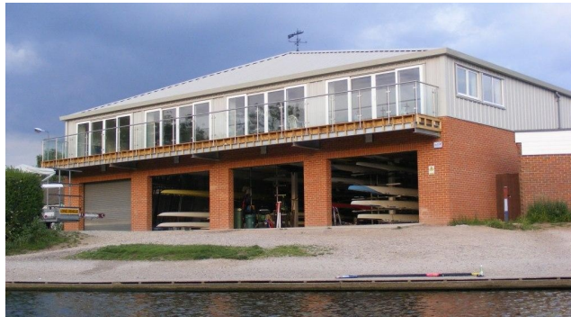
Balcony in place
